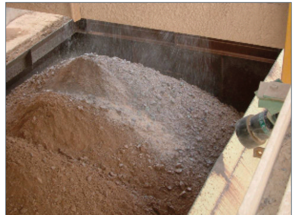
RAIL TRUCK LEVEL FOR WATER SPRAY CONTROL
